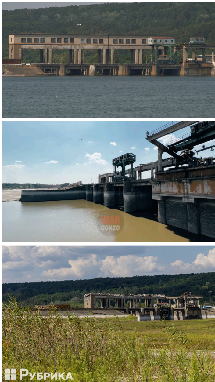
Figure 11: Oskil Dam facing the Oskil Reservoir in various stages of damage. From top to bottom: 2017; May 21, 2022; August 31, 2023.
